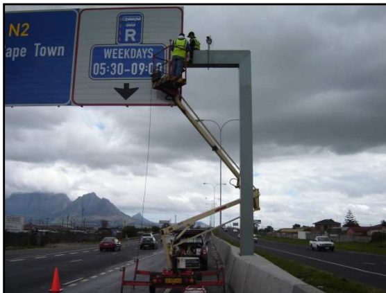
Installation of the ANPR cameras performing the automatic enforcement of the Bus lane
